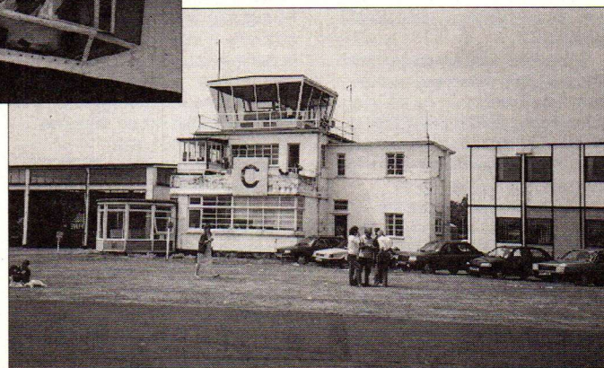
Control tower & fire station at Cranfield
